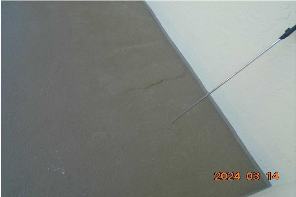
Figure 9. Surface spall at walkway 207.
