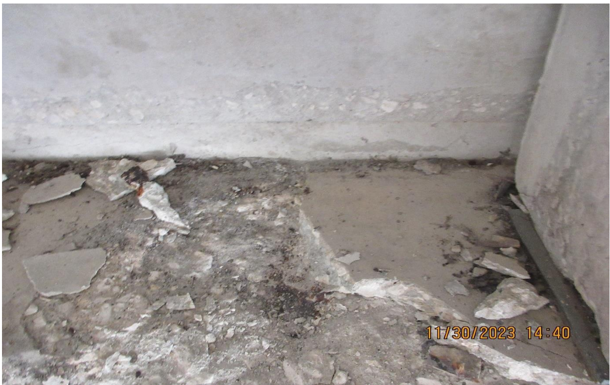
Figure 28. Spall was discovered at the top of the garage beam near the tee bearing point.
