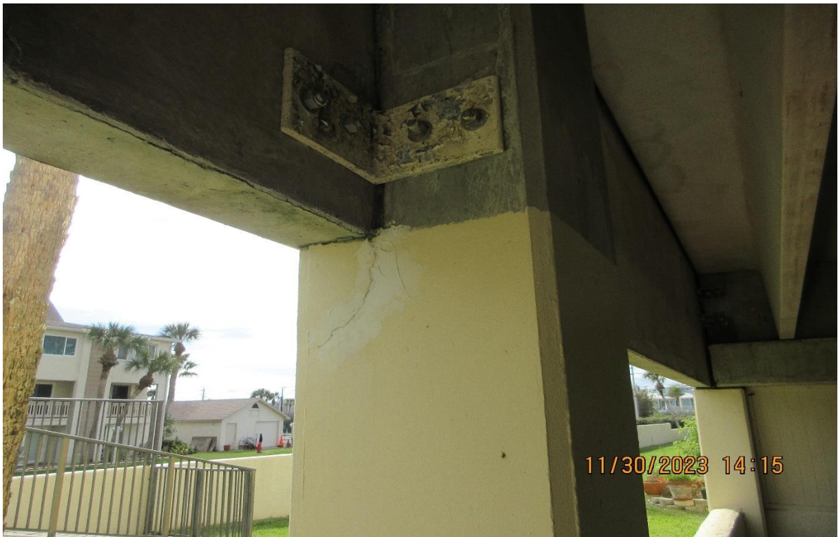
Figure 26. Column spall at south end of the garage.
