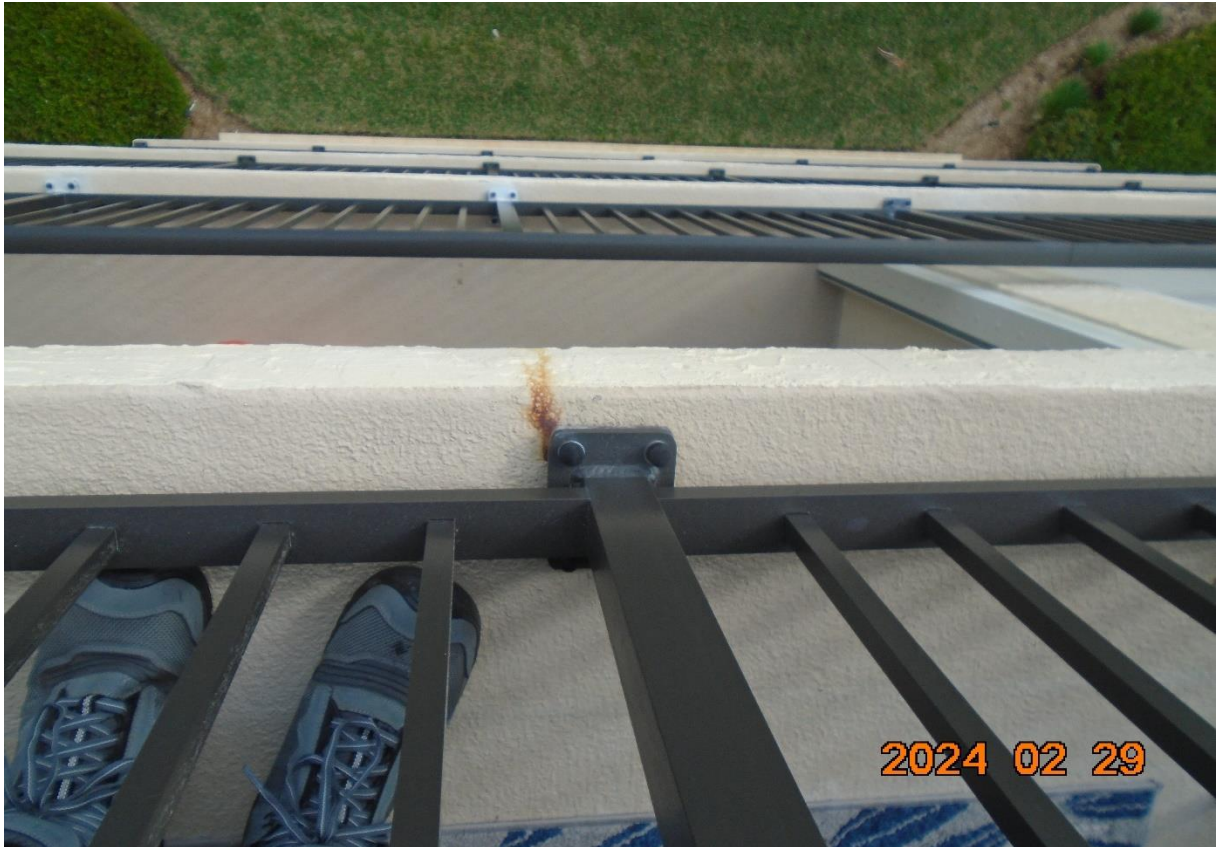
Figure 189. Example of a corroding anchor to be replaced under miscellaneous fastener Line Item of the budget.
