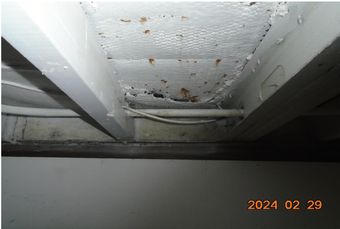
Figure 2. 202 living room east wall severely corroded framing and metal lath condition.
