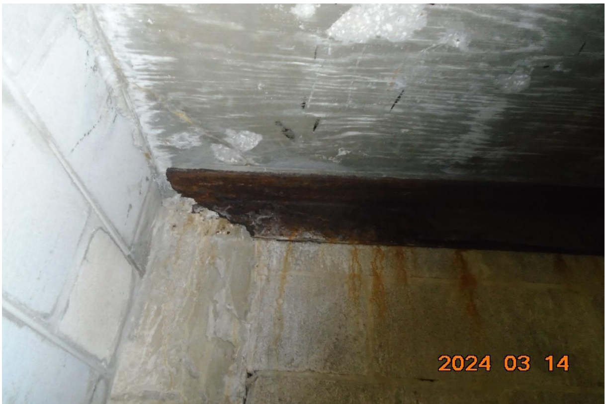
Figure 14. Generator room ledger angle corroded to failure.
