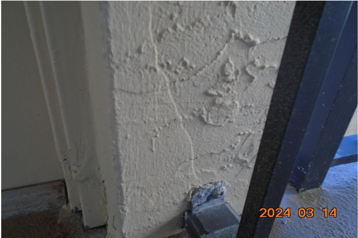
Figure 13. 2 nd floor north stairwell door jamb spall and rail receptor anchor failed from oxidation.
