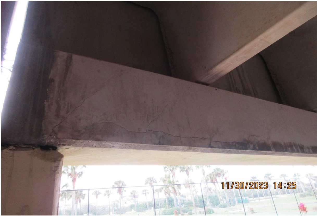
Figure 27. Garage west elevation perimeter beam spalled.
