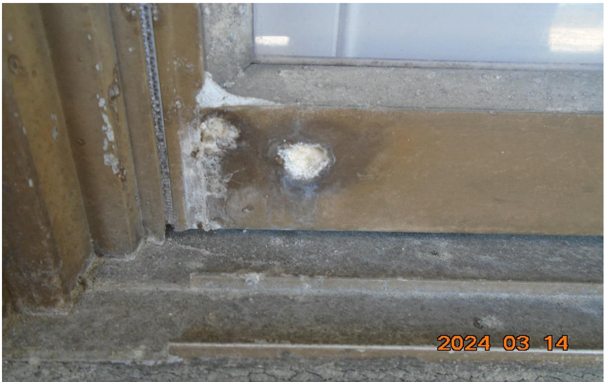
Figure 18. 103 walkway window reached useful life of structural connections.
