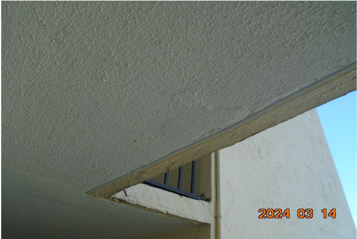
Figure 11. Edge spall overhead outside 204 entry door.
