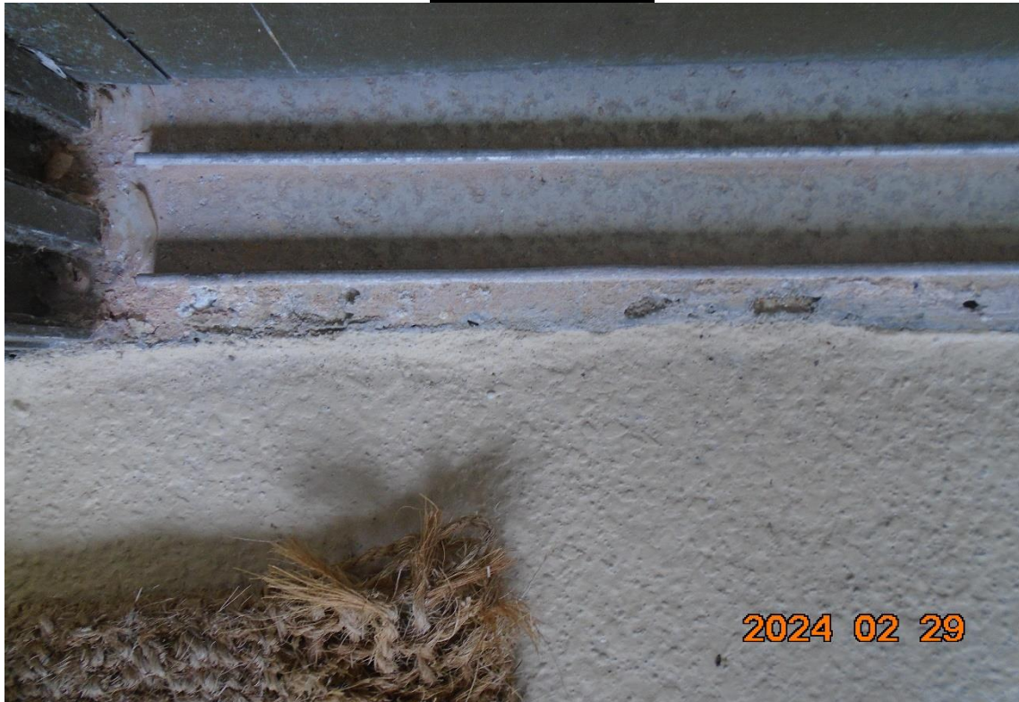
Figure 1. 306 sliding glass door threshold oxidized condition replacement is required to mitigate the water intrusion.
