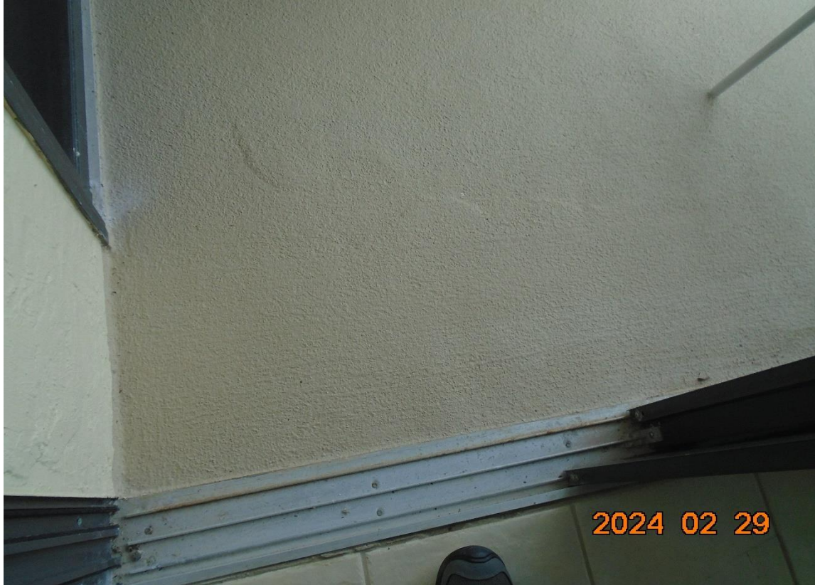
Figure 3. Example of a surface spall at 501 balcony.
