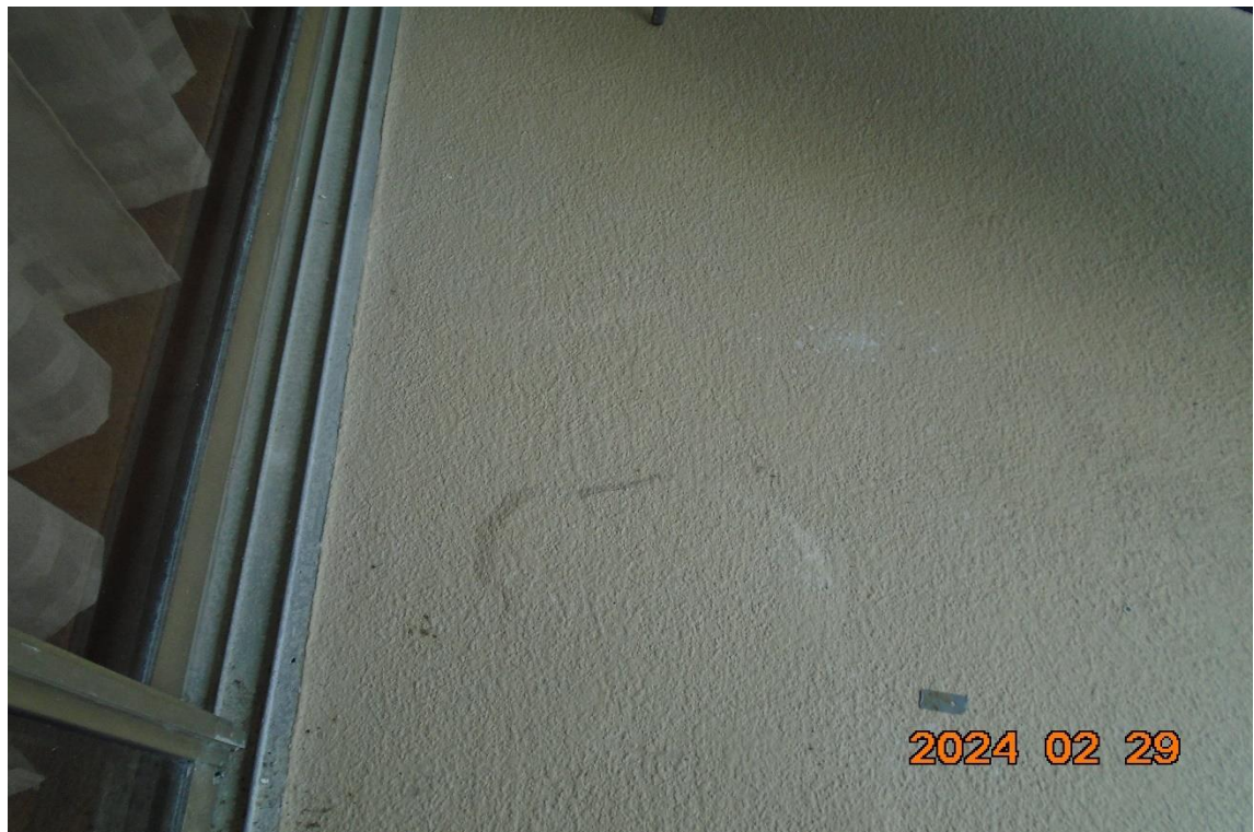
Figure 4. 504 balcony surface spall.
