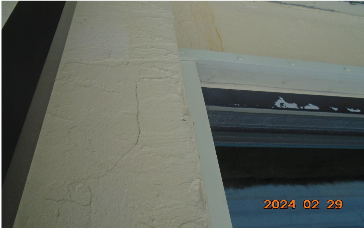
Figure 7. Example of a column spall outside 302 balcony.
