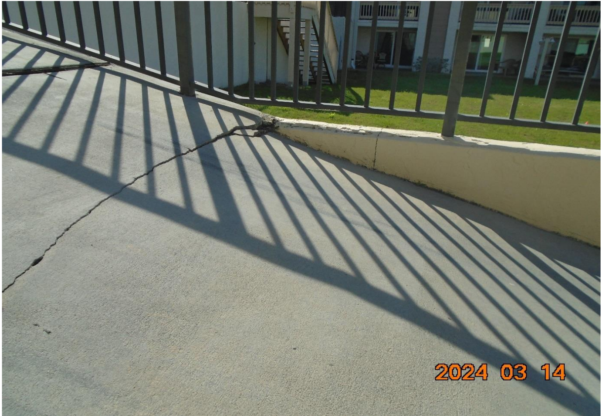
Figure 177. South elevation service ramp erosion and deflection with masonry cracking in walls.
