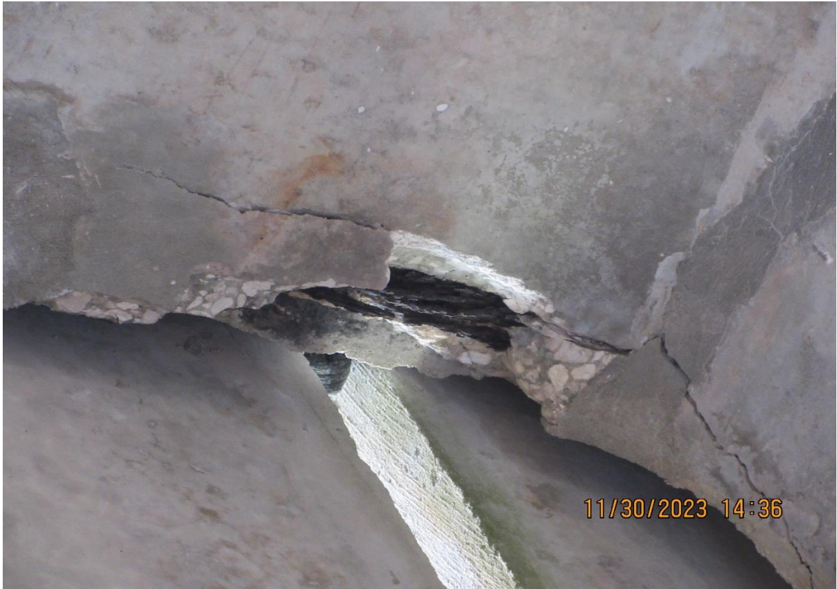
Figure 23. Example of double tee plate spall in garage.
