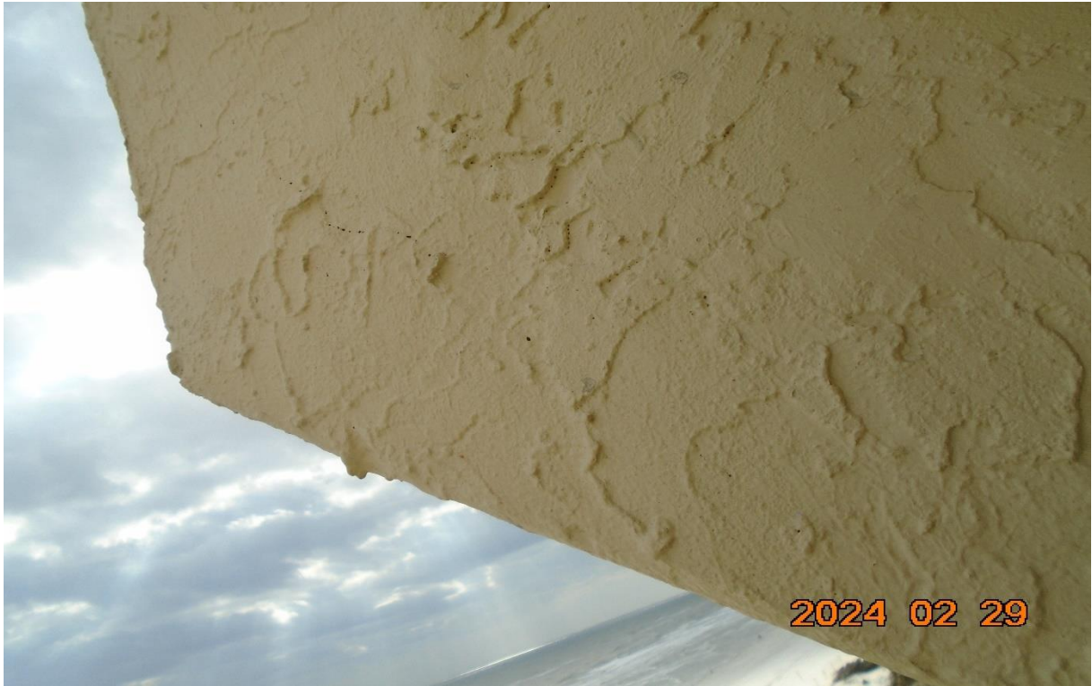
Figure 5. Roof parapet spall above 505 balcony.
