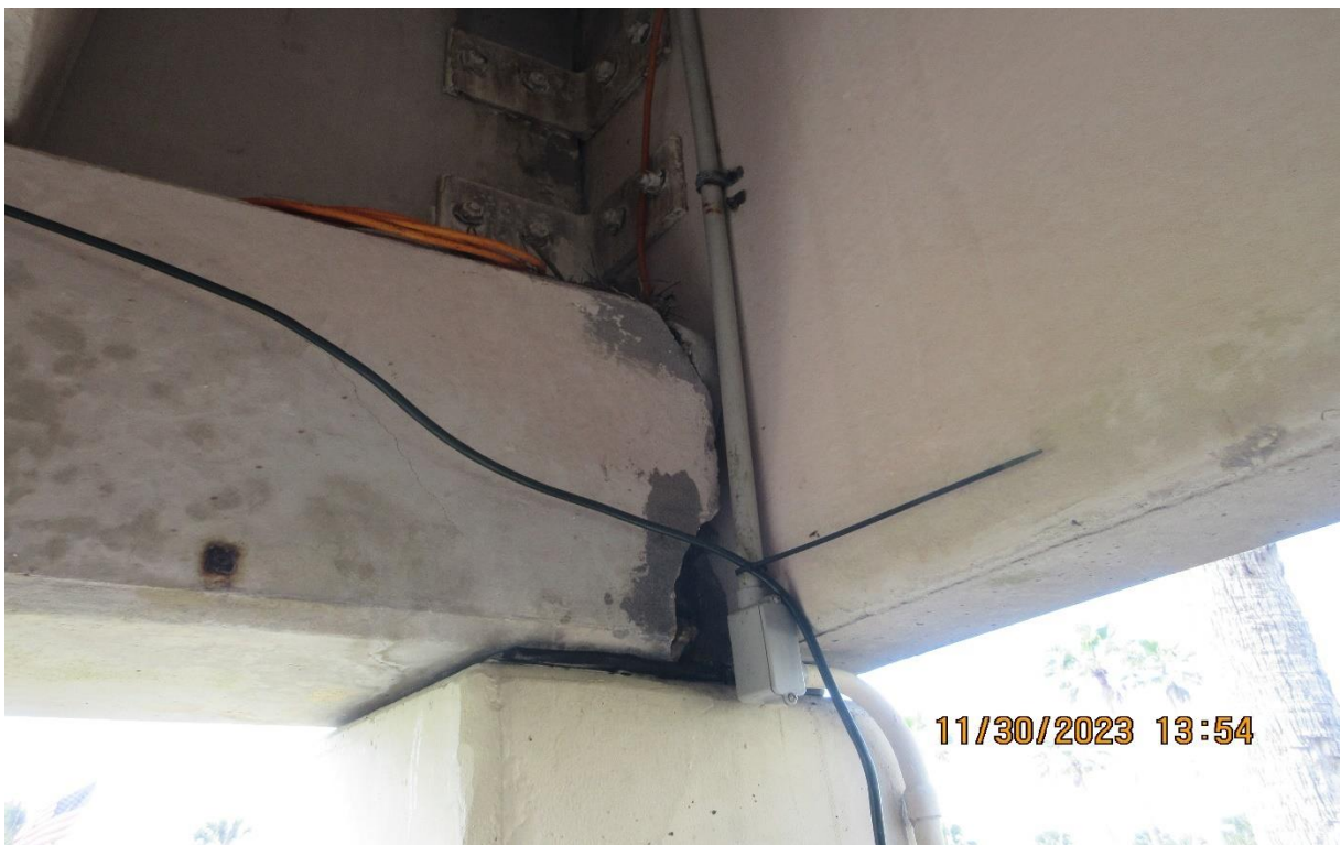
Figure 24. Example of garage perimeter beam end spall.
