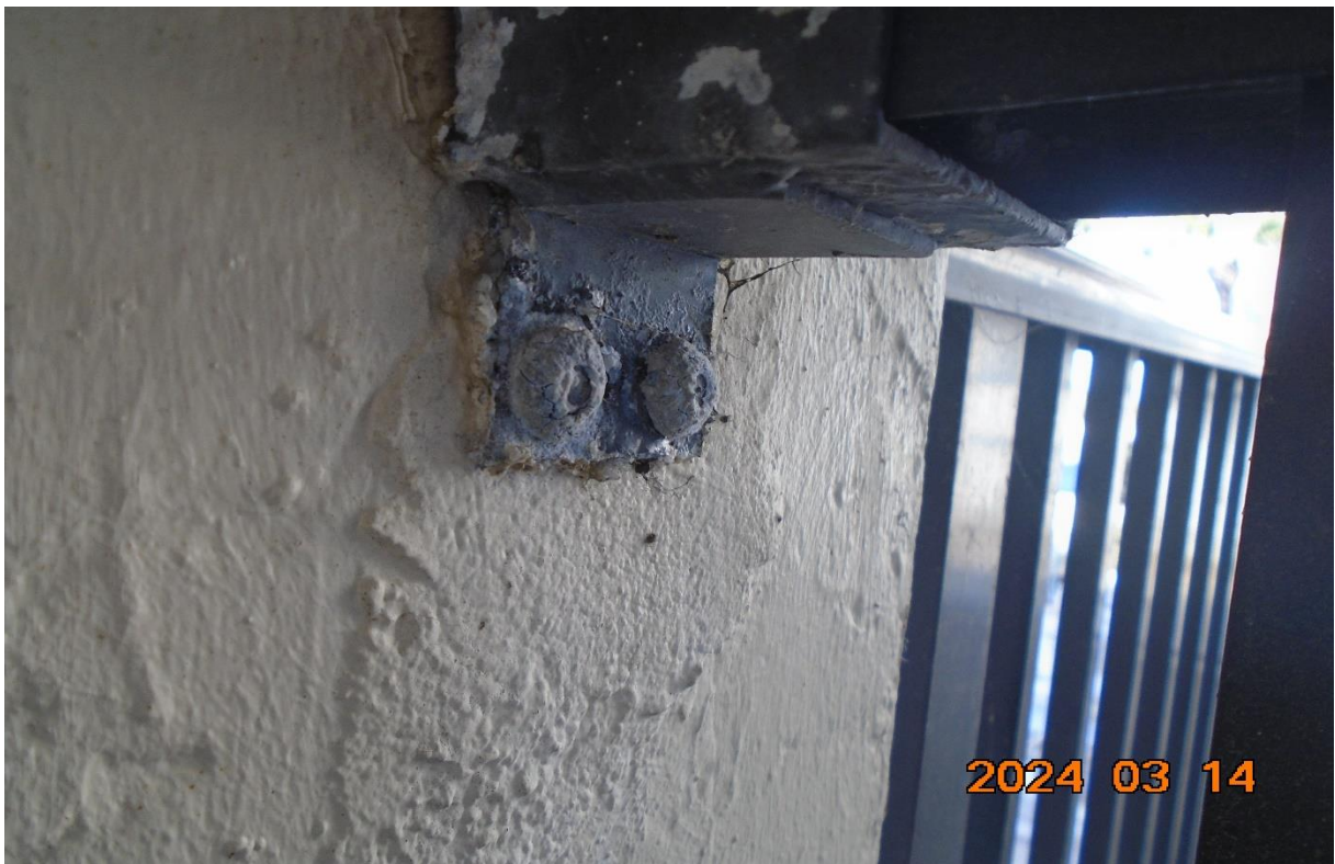
Figure 22. Example of oxidizing aluminum fasteners at walkway railing wall receptors.
