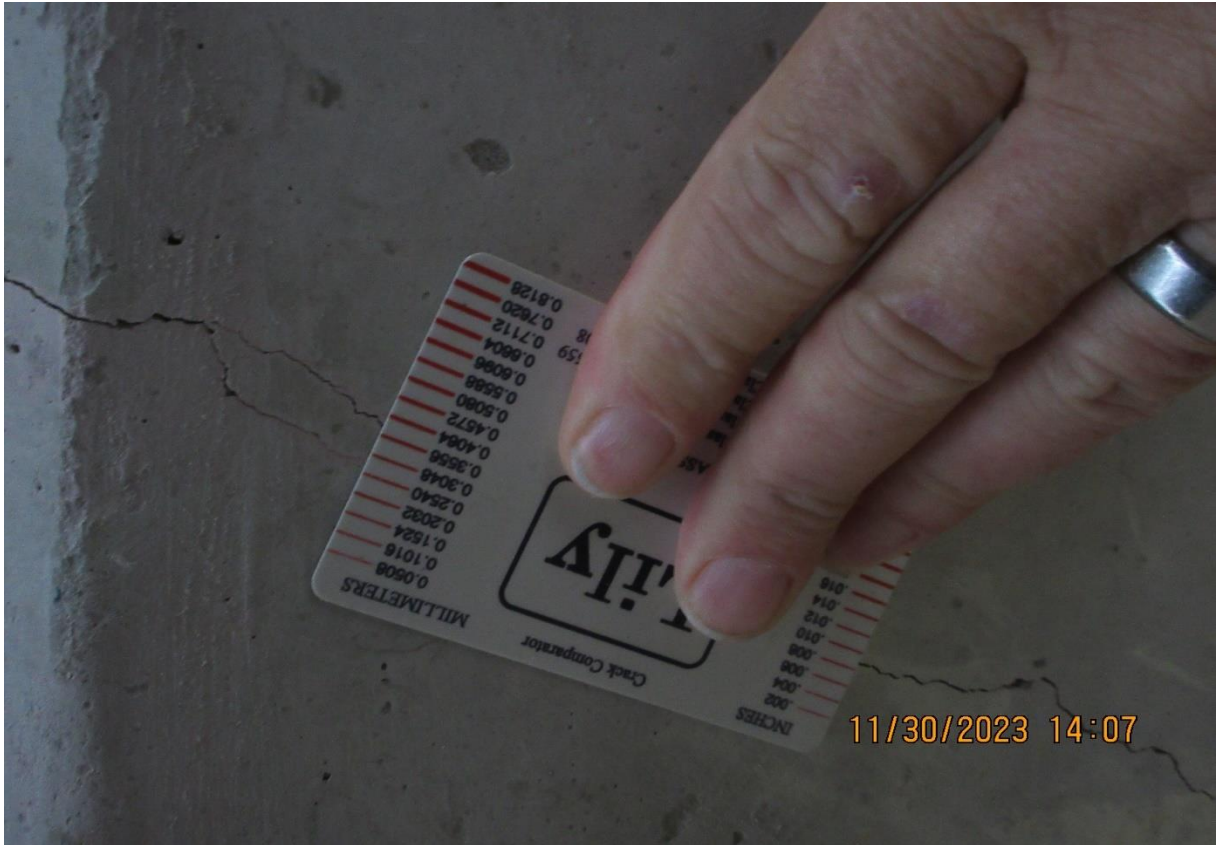
Figure 25. Example of garage perimeter beam cracks evaluated for diameter.
