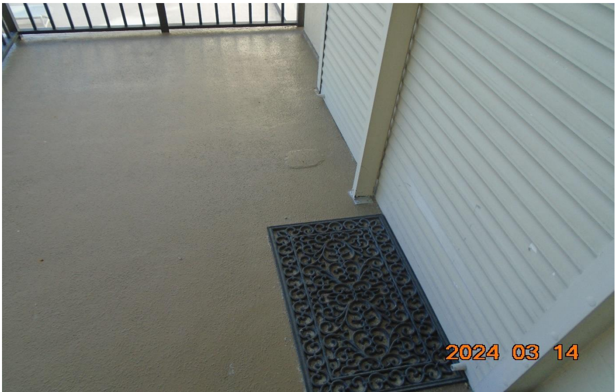
Figure 12. Unit 201 walkway balcony surface spall.
