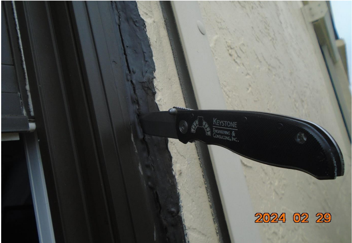
Figure 21. Example of many witnessed unsealed window and door assemblies.
