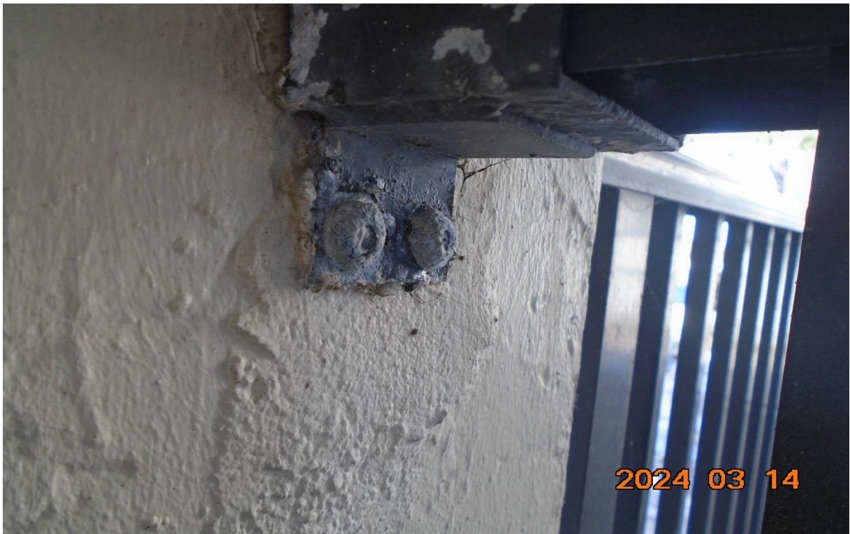
Figure 20. Example of oxidizing aluminum fasteners at walkway railing wall receptors.
