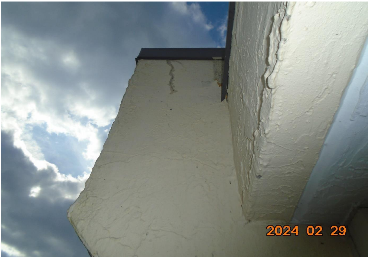
Figure 6. Parapet spall where coping cap may be impacted. `
